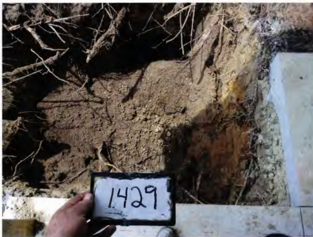
Picture 2: UST 1429 Albatross excavation.
